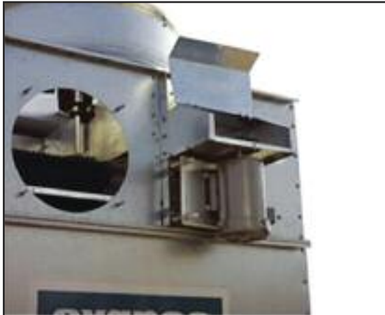
External Motor Mount (with swing away cover)
