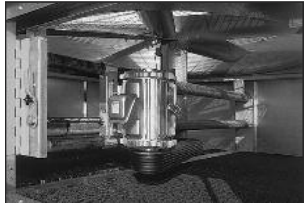
Motor Base Assembly
