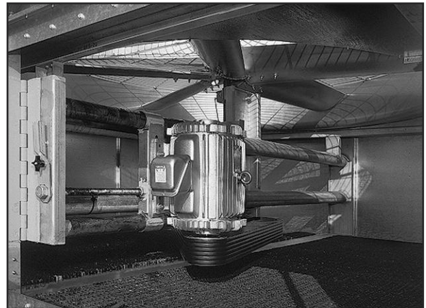
Motor Base Assembly
