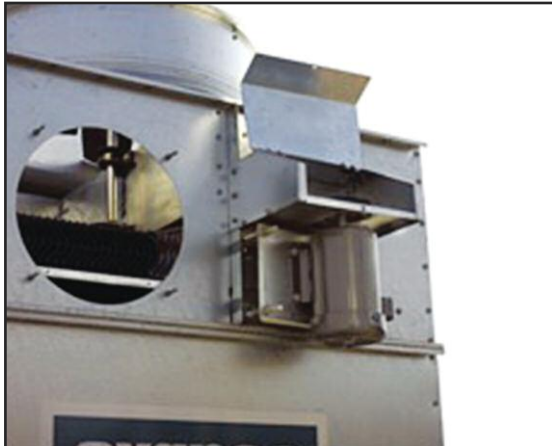
External Motor Mount (with swing away cover)
