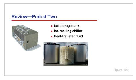
Period Two discussed the three components of a glycol-based ice storage system that are different from a conventional chilled-water system: the ice storage tank, the ice-making chiller, and a heat-transfer fluid that remains liquid at temperatures lower than the freezing point of water.
