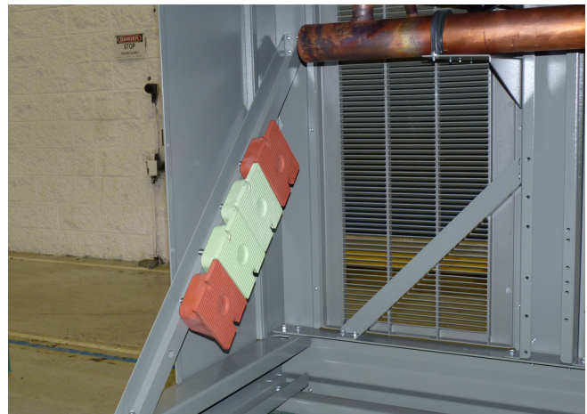
Figure 4. Elastomeric isolators attached for shipping
